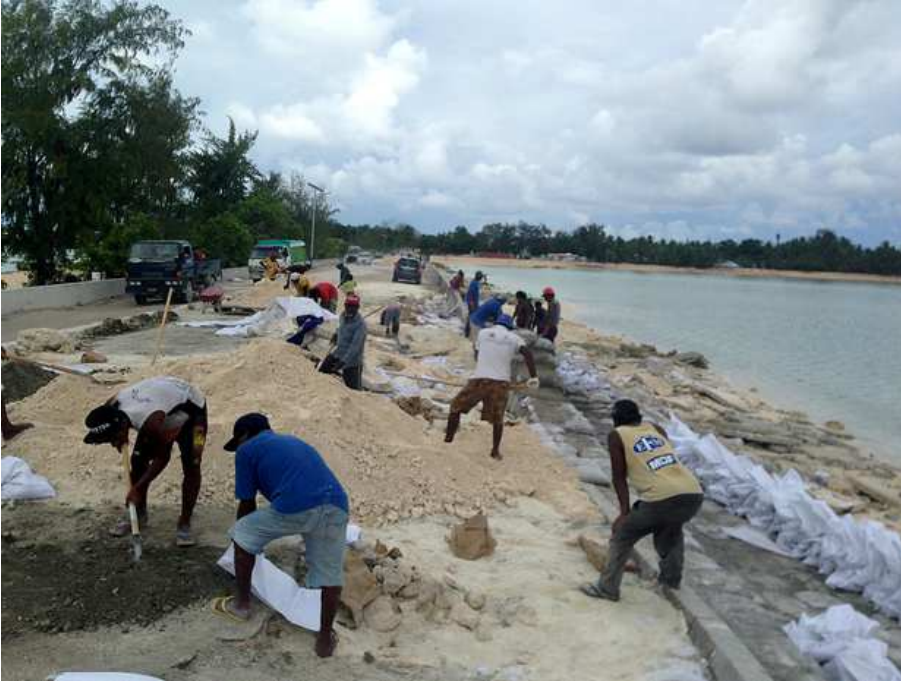
Sand bagging the beach to stop erosion in Tarawa, Kiribati. Photo: Supplied
