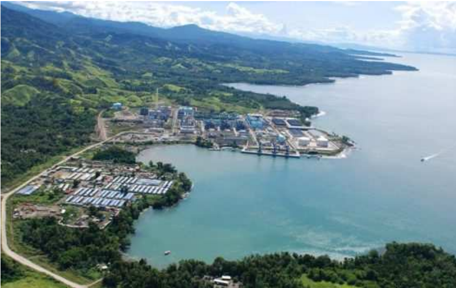
MCC's Basamuk Refinery in Madang pumps waste from the Ramu mine directly into the ocean
