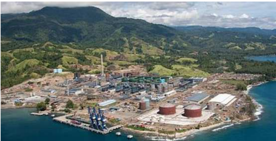
The Basamuk refinery which has been closed down until remedial steps are taken
