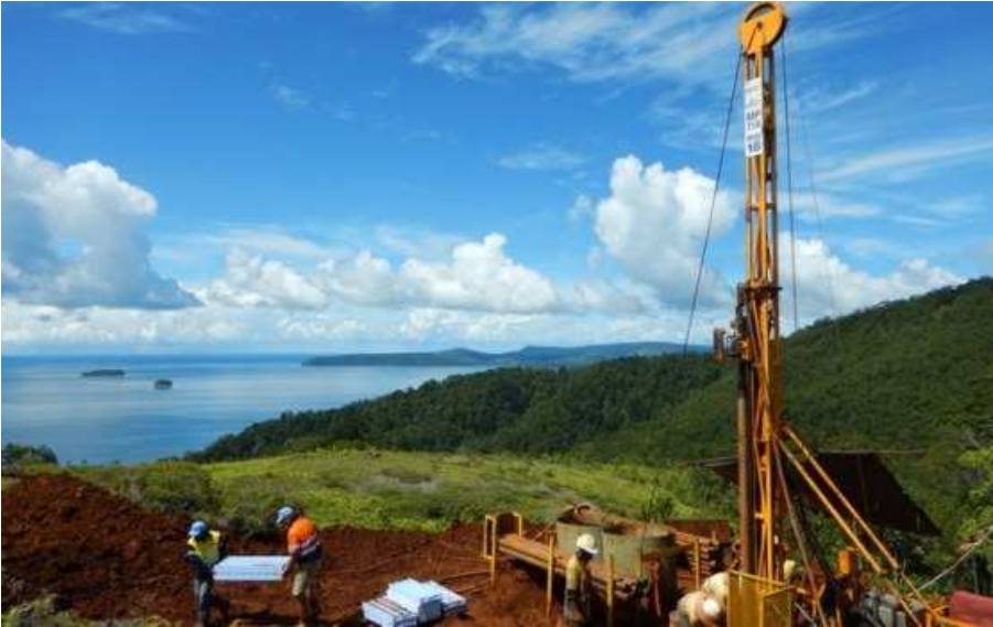
Axiom drilling activity on Isabel Nickel Project.
