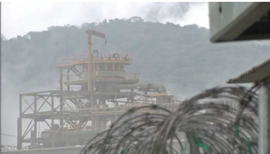
Abandoned Gold Ridge mine processing plant. (Stefan Armbruster SBS)
