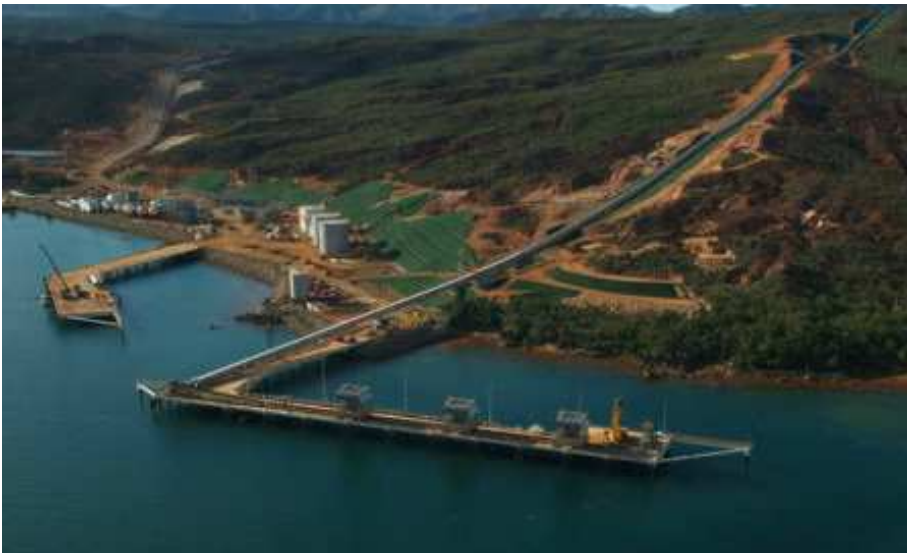
Port of New Caledonia's Vale nickel plant Photo: supplied
