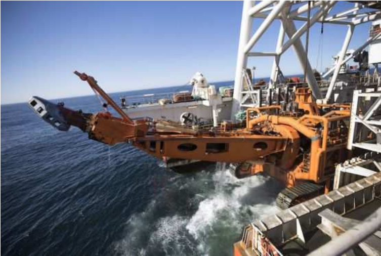
The giant subsea "crawler" tractor is lowered into the ocean from the deck of the Mafuta.
