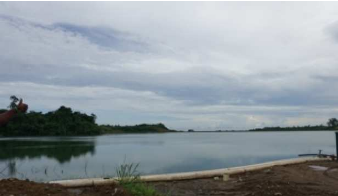
The tailings dam at the Gold Ridge mine. Credit: Matthew Allan, Australian National University.
