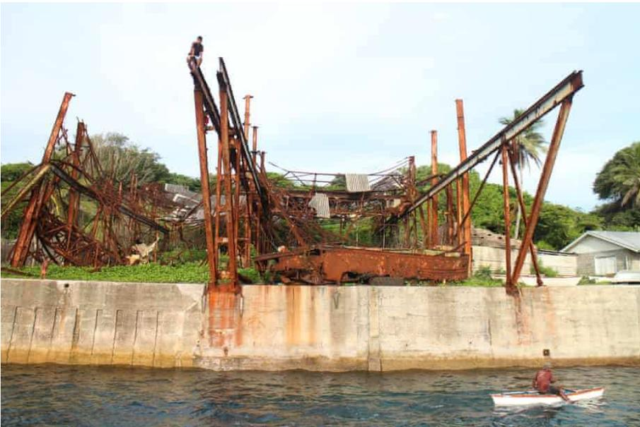
The old cantilever that used to load phosphate on to ships. Photograph: Janice Cantieri
