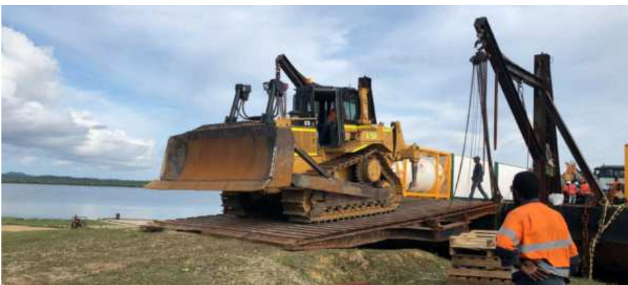
Construction has started at the Woodlark gold project. Photo: Geopacific Resources
