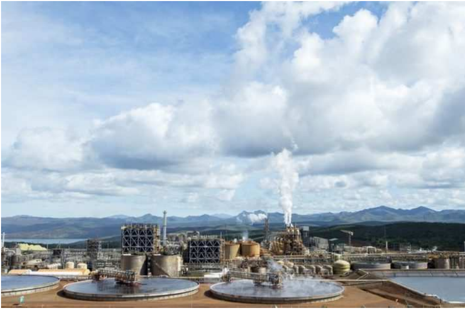
A photo taken on May 27, 2015 shows Brazilian Vale's nickel processing plant of Goro in southern New Caledonia. Photo: AFP PHOTO / FRED PAYET
