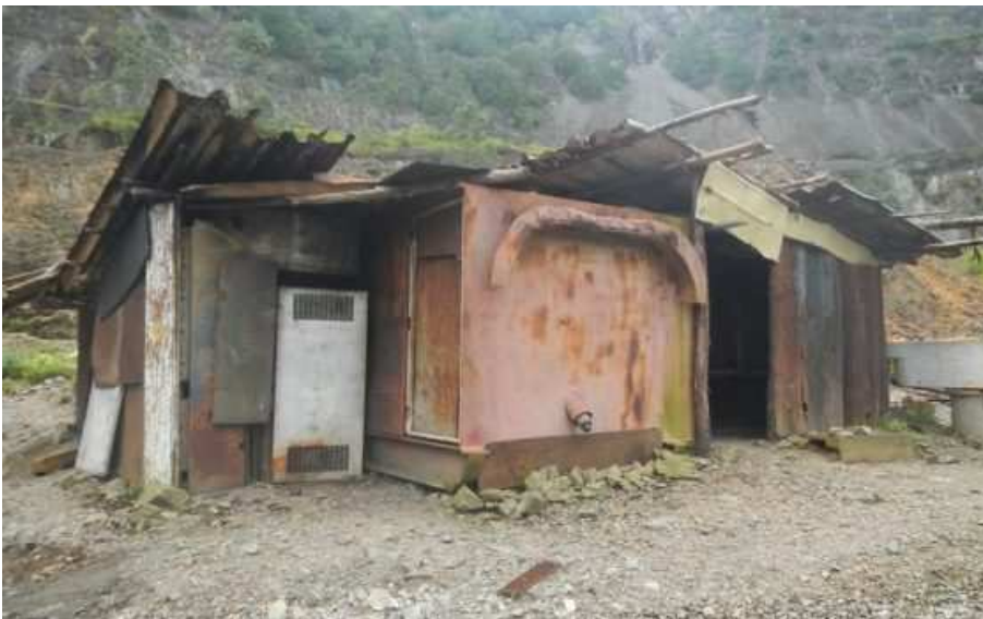
An abandoned building at Panguna mine site in Bougainville
