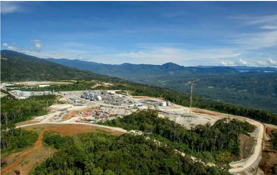
Exxon Mobil PNG's Hides gas conditioning plant Photo: Richard Dellman
