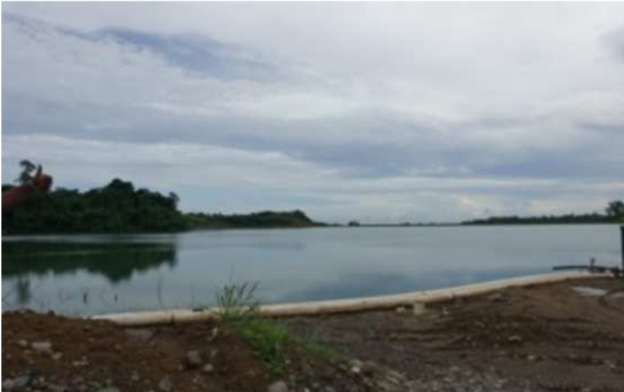
The over-full tailings dam facility at the Gold Ridge Gold Mine on Guadalcanal in Solomon Islands in January 2015. Photo: copyright Dr Matthew Allen – ANU
