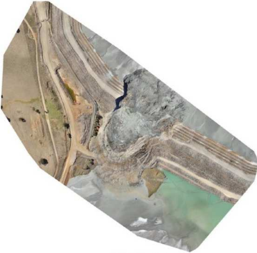
A close-up of the dam wall breach.
