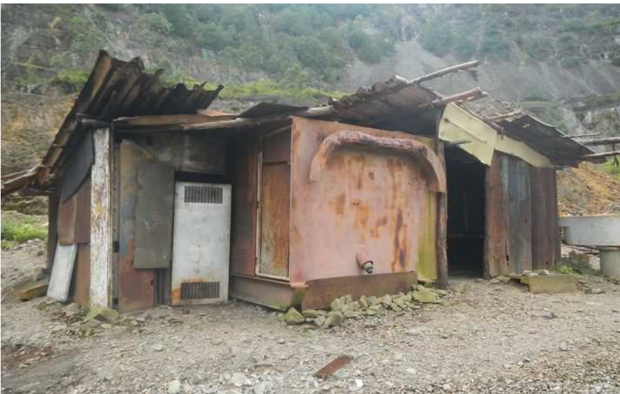
An abandoned building at Panguna mine site in Bougainville Photo: supplied
