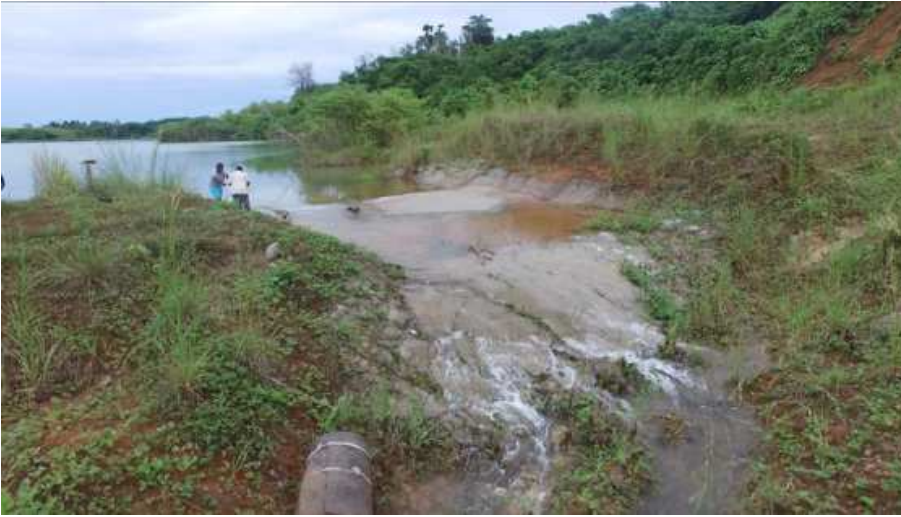
Water spills over the Gold Ridge tailings dam wall
