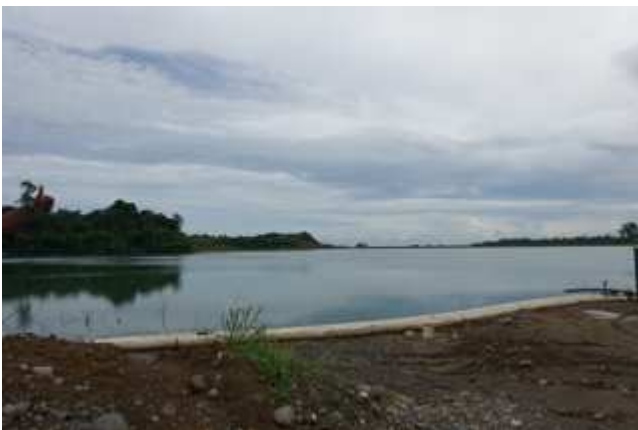
The over-full tailings dam facility at the Gold Ridge Gold Mine on Guadalcanal in Solomon Islands. January 2015. At the time this was captured the water level was one metre from the brink with 3 months to go in the wet season. Photo: copyright Dr Matthew Allen - Australian National University
