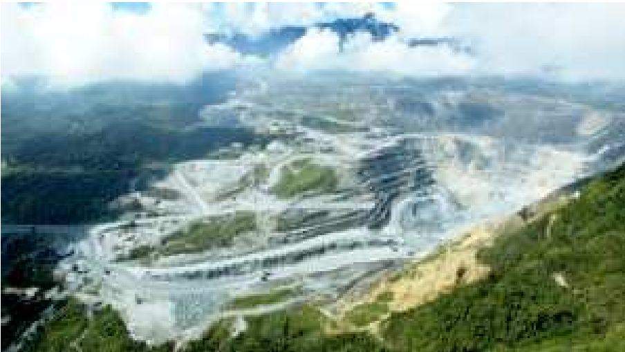
The Porgera mine in Papua New Guinea. (Image courtesy of Barrick Gold .)
