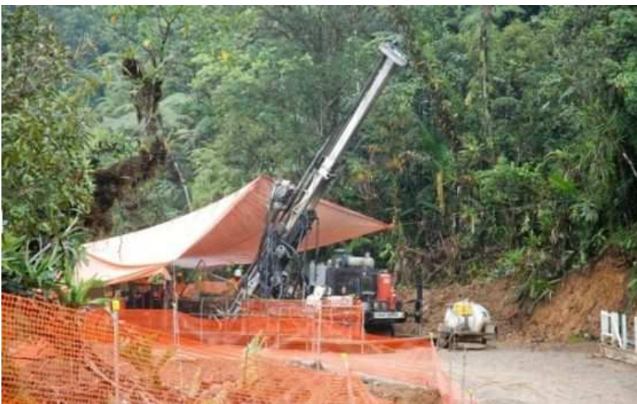
A drill pad site.
