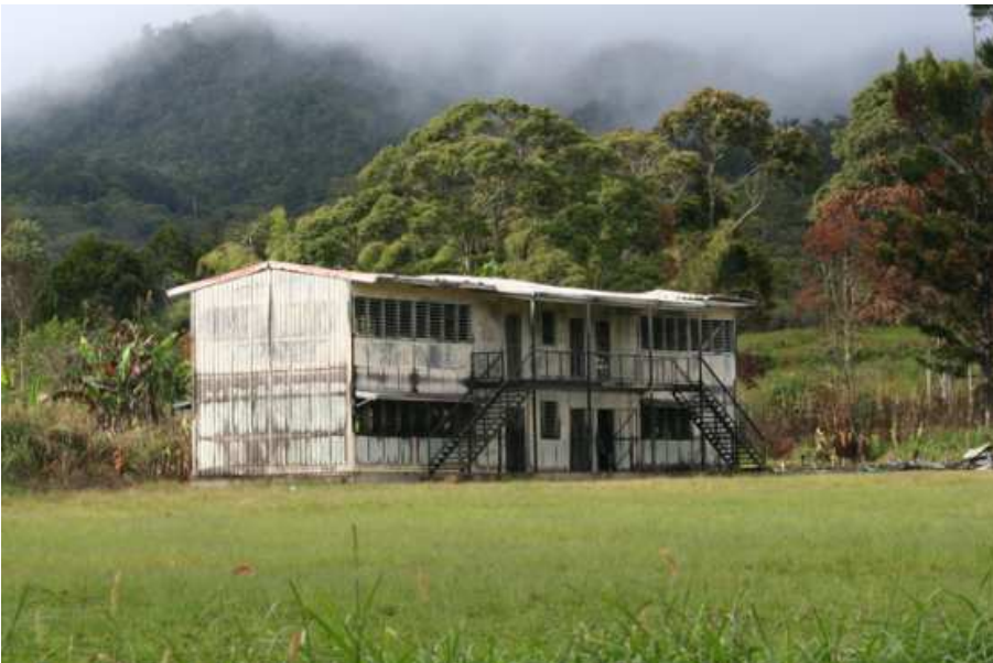
A school burnt out as a result of tribal conflict in Papua New Guinea's Hela province. Photo: RNZ / Johnny Blades
