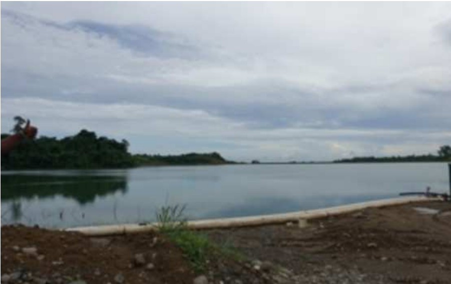
The over-full tailings dam facility at the Gold Ridge Gold Mine on Guadalcanal in Solomon Islands in January 2015. Photo: copyright Dr Matthew Allen - Australian National University
