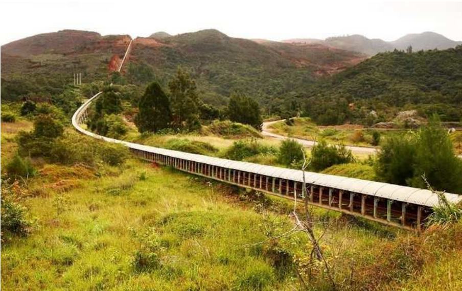
The conveyor belt at the Kouaoua mine. Photo: SLN
