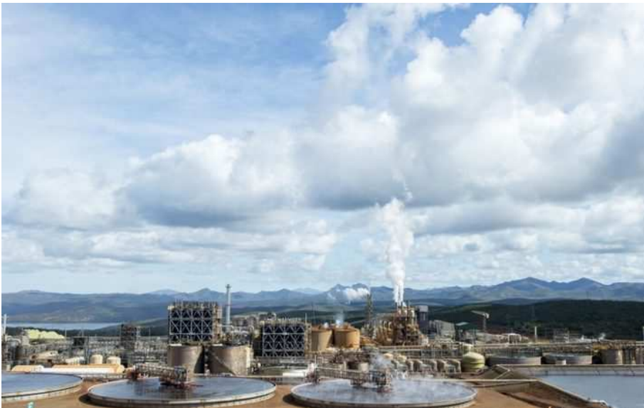
Vale's plant in Goro Photo: AFP PHOTO / FRED PAYET
