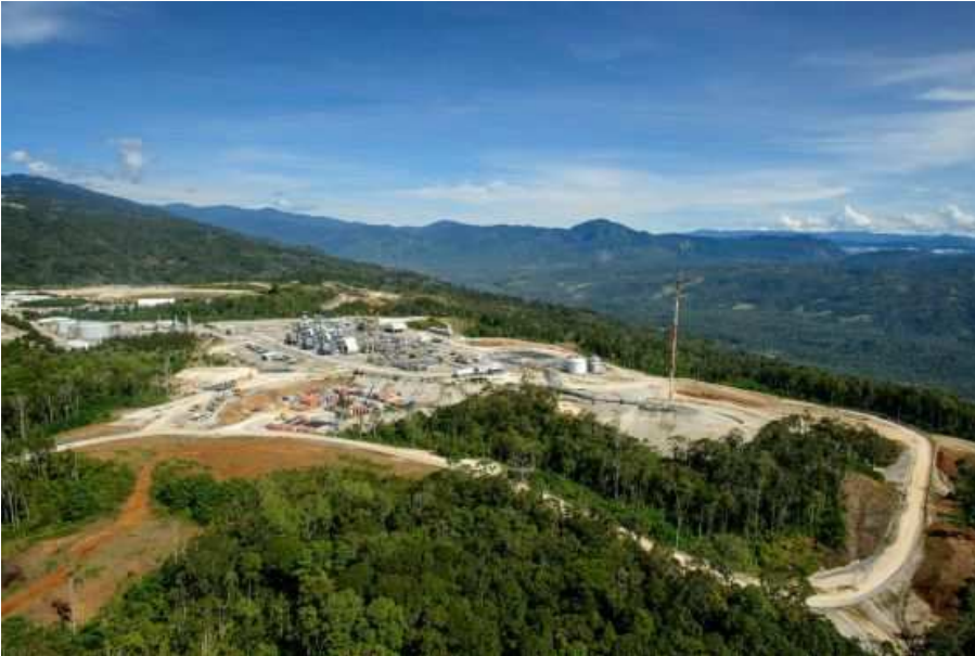
Hides Gas Conditioning Plant in Papua New Guinea. Photographer: Richard Dellman via Exxon Mobil Corp.
