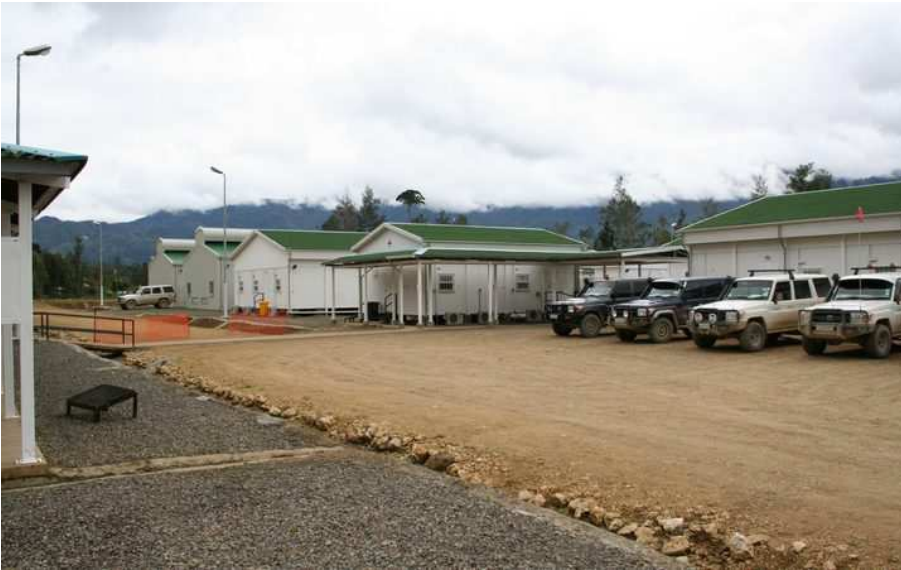
LNG Project site in Papua new Guinea's Hela Province. Photo: RNZ / Johnny Blades
