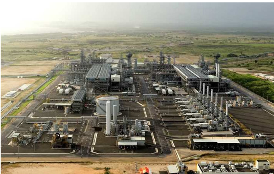
Exxon Mobil PNG's LNG plant near Port Moresby Photo: (C)2014 {Richard Dellman/AdvantagePNG}, all rights reserved
