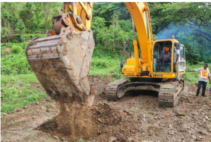
Acting Prime Minister and Minister for Industry, Trade and Tourism Faiyaz Koya breaks ground marking the beginning of the civil works on November 17, 2017. Photo: DEPTFO
