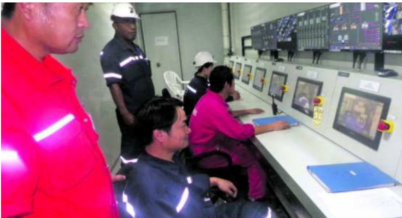
Chinese engineers at the control centre at the new power house at Vatukoula Gold Mines. Photo: Karalaini Tavi
