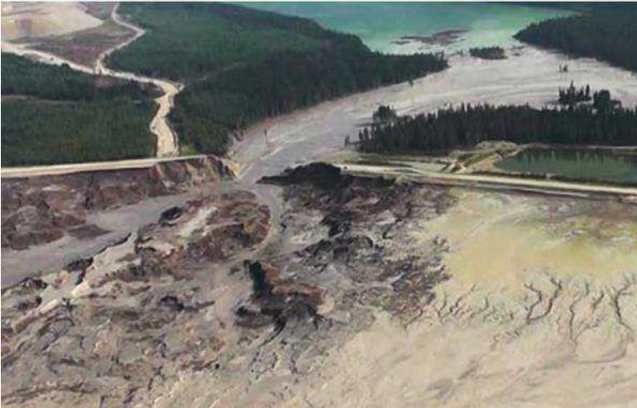
The Imperial Metals Mount Polley gold and copper mine tailings dam disaster in British Columbia, Canada, dumped 24 million cubic meters (more than 31 million cubic yards) of mine waste and sludge into neighboring Lake Polley and polluting the Hazelton Creek watershed. Photo courtesy of the Multinationals Observatory
