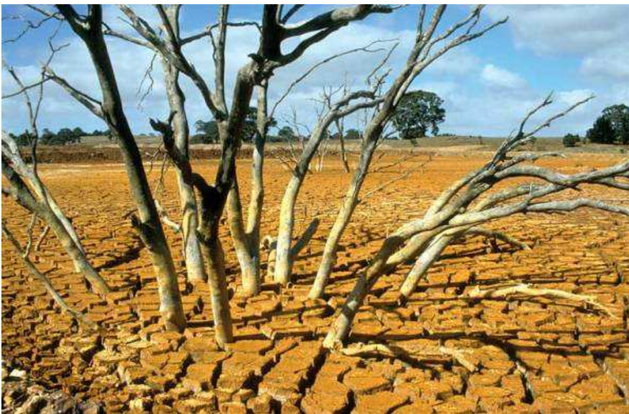
Dry bed of the tailings dam at the Brukunga Pyrite Mine east of Adelaide in the Mount Lofty Ranges, South Australia. The mine was closed in 1972 and this photo comes from 1992. In 1974, a severe storm resulted in the retention ponds overflowing into nearby Dawesley Creek with water quality impacts occurring downstream. Tailings dams continue to be environmental hazards long after mine closures. Photo courtesy of CSIRO ScienceImage licensed under CC BY-NC-ND 4.0
