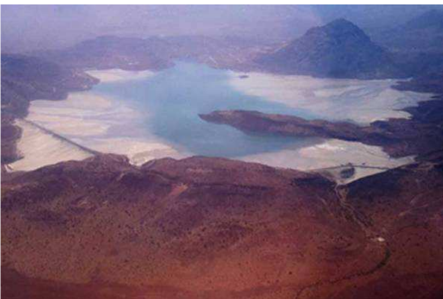
La Tortolas tailings dam high in the Andes Mountains of Chile. The dam was built in a seismically active area, but is designed to resist earthquakes. Photo by Lodecop licensed under the Creative Commons Attribution-Share Alike 3.0 Unported license
