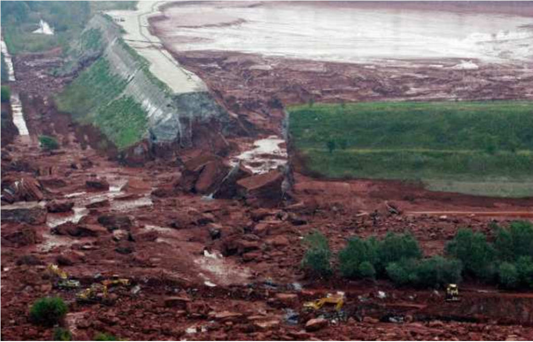
An aerial photo taken Tuesday, Oct. 5, 2010 shows the ruptured wall of a red sludge reservoir of the Ajkai Timfoldgyar plant in Kolontar, 160 km (100 mi) southwest of Budapest, Hungary. Note the excavators at bottom to give a sense of scale. Image Credit: AP Photos/MTI, Gyoergy Varga
